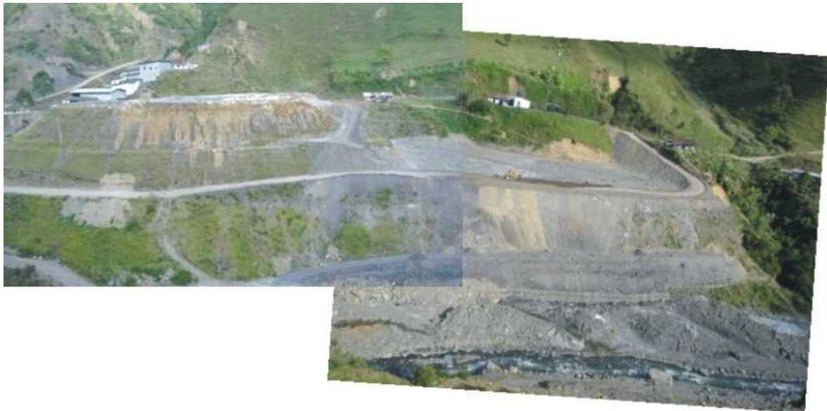
Figure 34. Repairs to the tailings impoundment, photo taken January 17, 2010.
