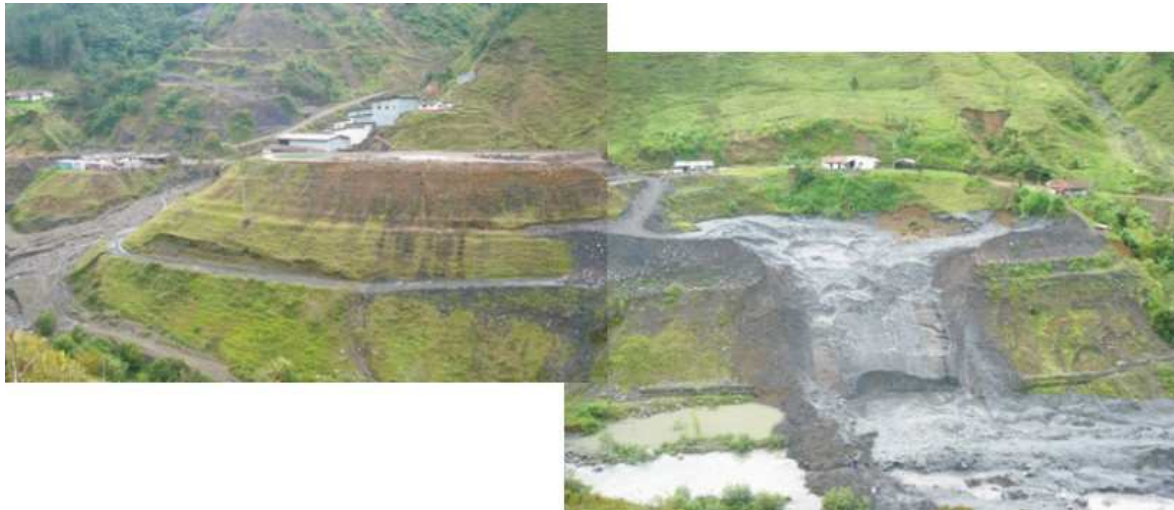
Figure 33. Tailings failure of August 13, 2009.
