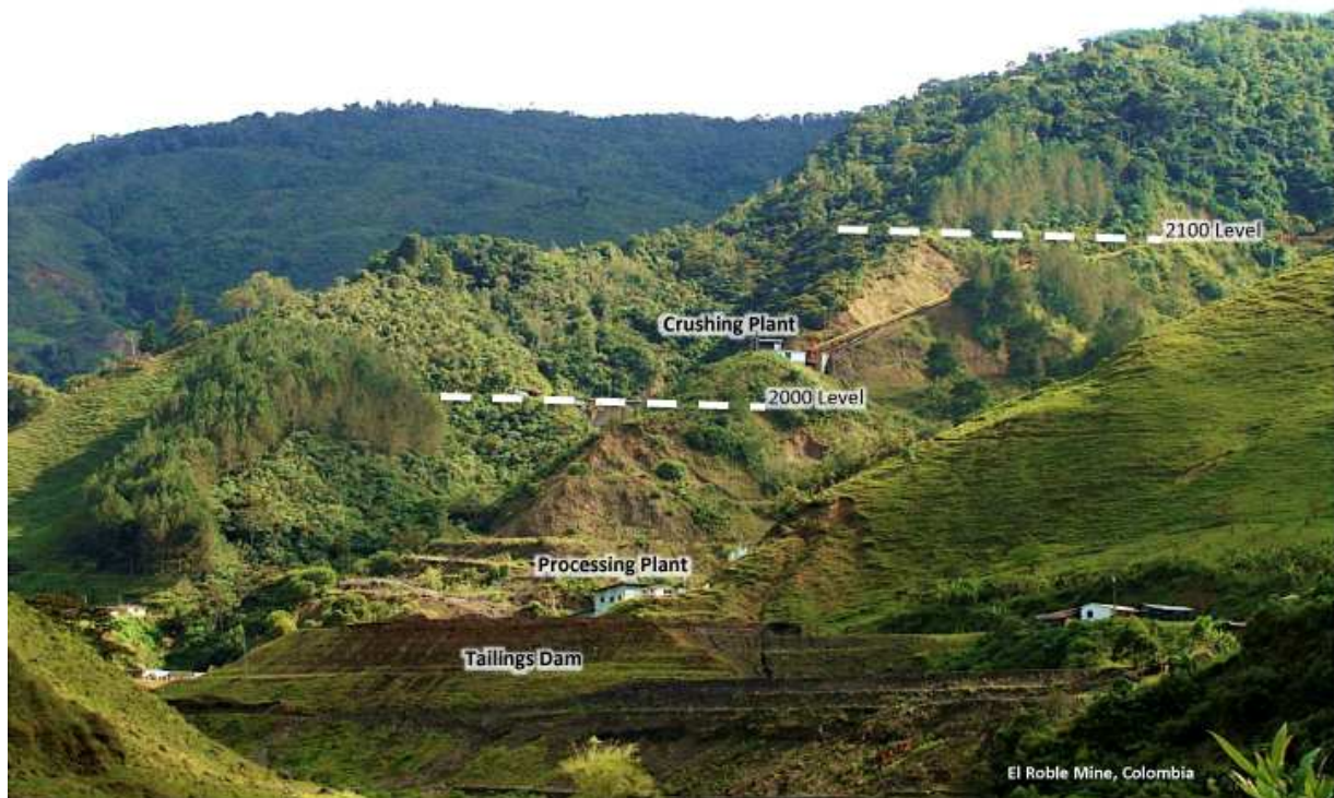
Figure 1 Overview of the El Roble mine site. The 2000m level tunnel is visible above the plant, which is located behind the tailings impoundment. The Atrato River, barely visible at the bottom of the photograph, flows north to south, towards the viewer. The original discovery outcrop is out of sight to the right, at the top of the ridge.
