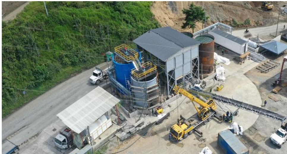
Figure 1 - El Roble, ITDS during Construction
